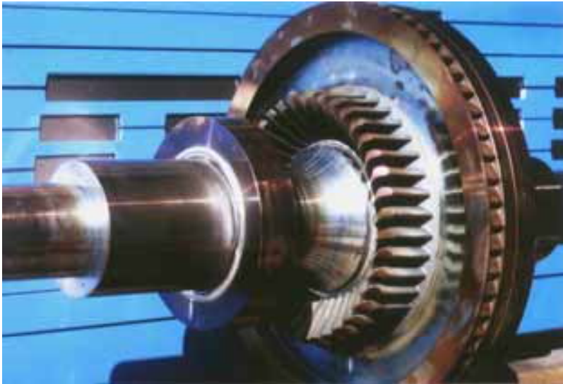
Fig. 255: Worn out parts of a turbine rotor are exchanged with new ones.
