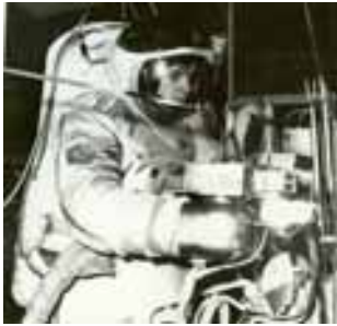
Fig. 1: Weld repairs to the MIR space station with a hand held EB gun.
