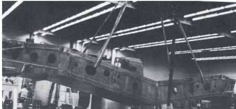
Fig. 139: Wing box of MRCA plane.
