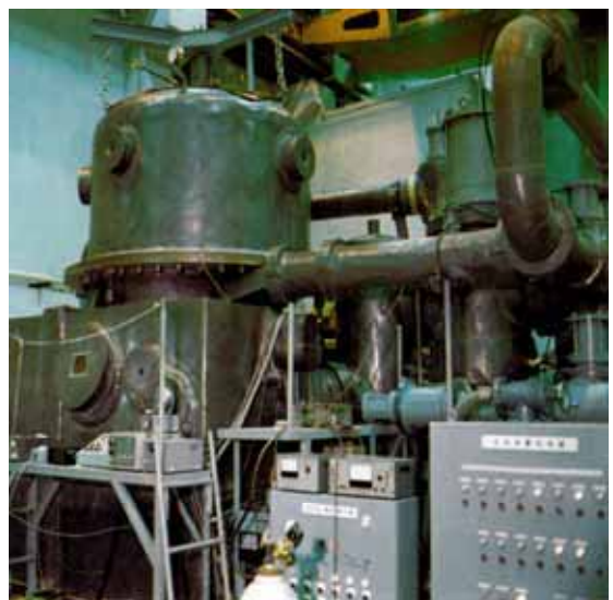
Fig. 92: In 1975 the voltage was increased to 300 kV, 100 kW [67].
