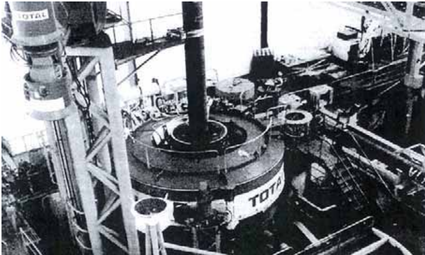
Fig. 39: Local vacuum machine for welding pipelines in the J position (1978).
